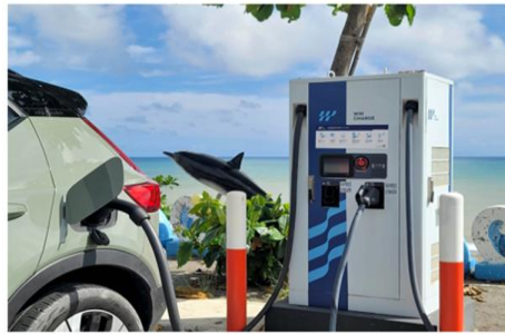
Charging Station Installation
